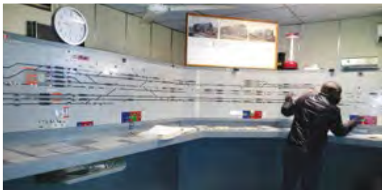
Above: The inside of the Train Control Room at the Elandsfontein Station in Gauteng, where one can get a bird's eye view of the Prasa railway route with all its railway stations from Pretoria to Johannesburg on the control panel. This is one of eight existing passenger train control rooms that will be consolidated into the single, high-tech super control centre at Kaalfontein. Middle: UNTU member Kabomo Mpho Lamola announces the trains on the intercom in the Elandsfontein Signal Cabin in Gauteng. As soon as the Gauteng Nerve Centre is fully functional, Kabomo will work from the Nerve Centre and will no longer be stationed at the Elandsfontein Station. Above right: Commuters waiting for a train to Pretoria to arrive at the Elandsfontein Station. Delays are on average up to 30 minutes due to the shortage of trains.
